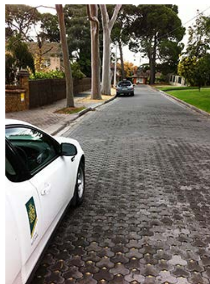
Permeable paving in Brookside Road, Springfield.
