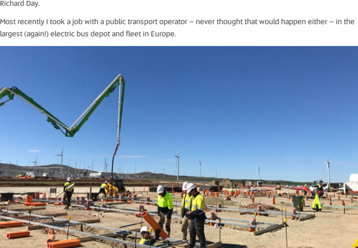
Image: Construction of the Hornsdale Power Reserve in regional South Australia
